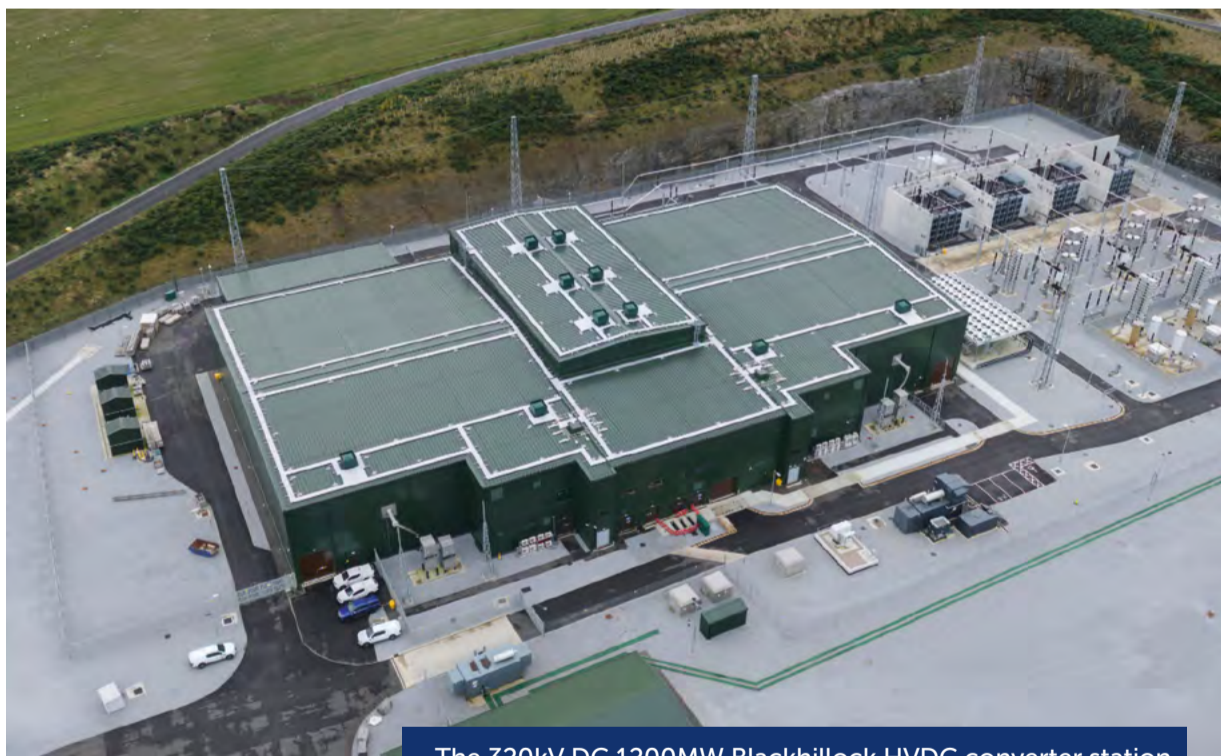
The 320kV DC 1200MW Blackhillock HVDC converter station
