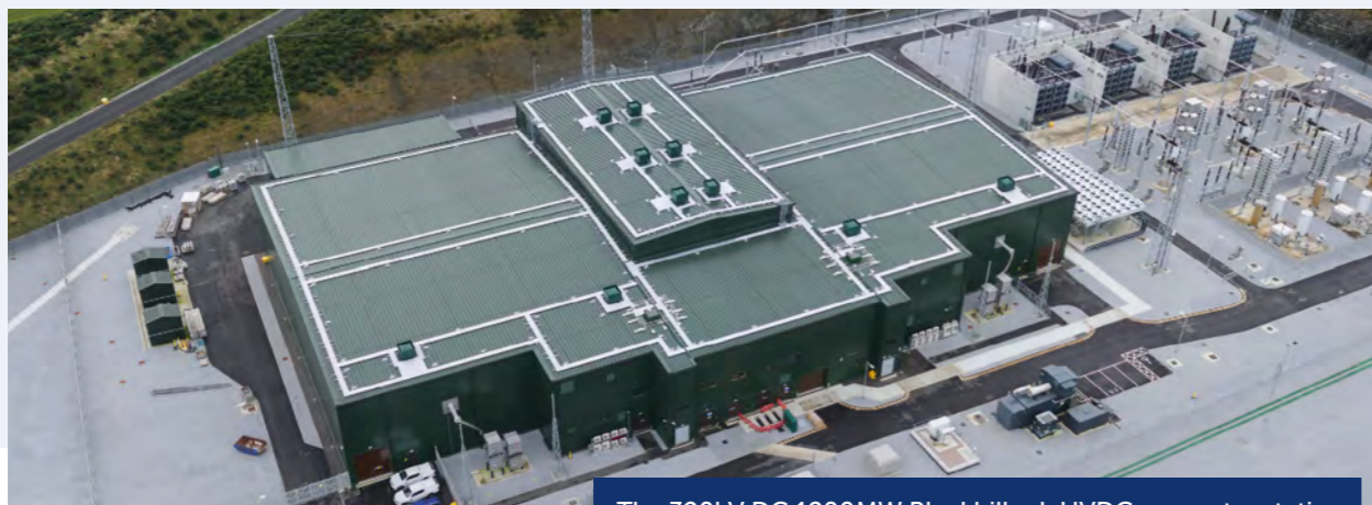
The 320kV DC 1200MW Blackhillock HVDC converter station
