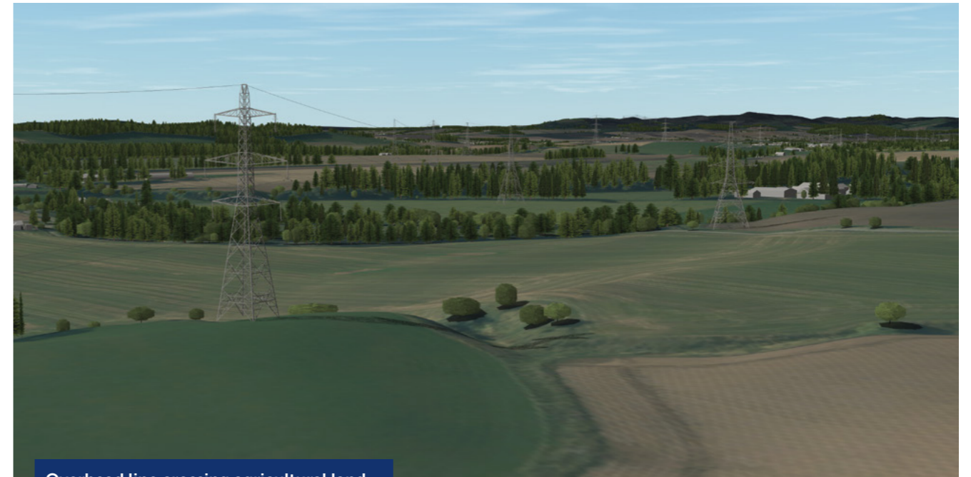
Overhead line crossing agricultural land
