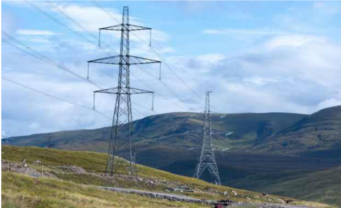
Plate 2.1 – Existing SSE400 Steel Lattice Tower Design
