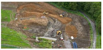
SSEN's Transmission's 132kV transformer replacement project adjacent to Lochay Power Station involves the construction of a new substation compound, including building to house indoor equipment.
