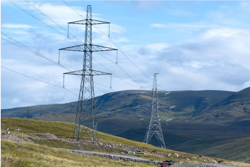
Plate 2.1 – Existing SSE400 steel lattice tower design
