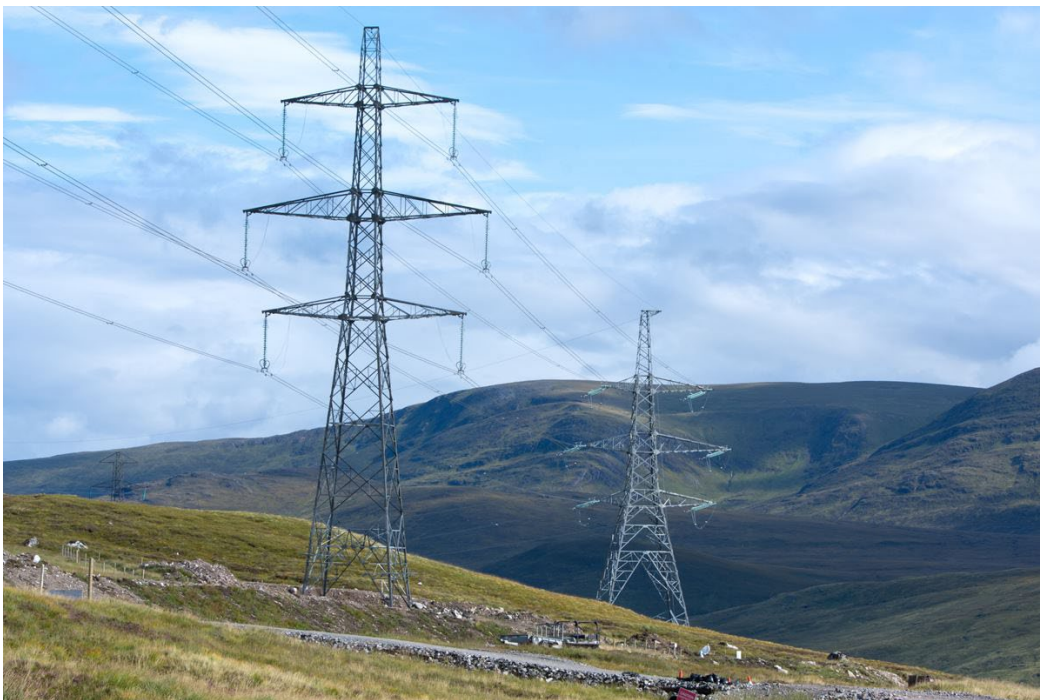
Plate 2.1 – Existing SSE400 steel lattice tower design
