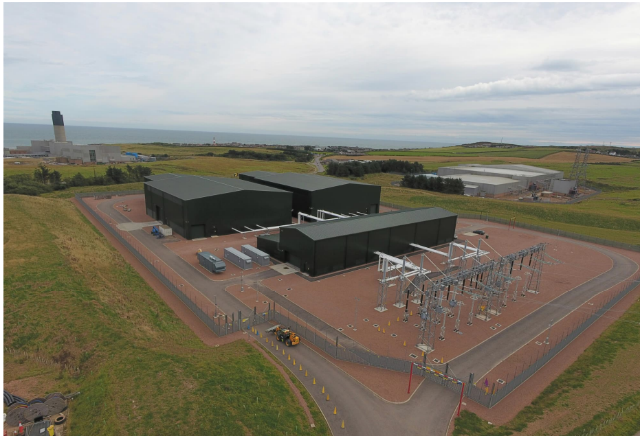
Plate 3-1 Example 400 kV Substation
