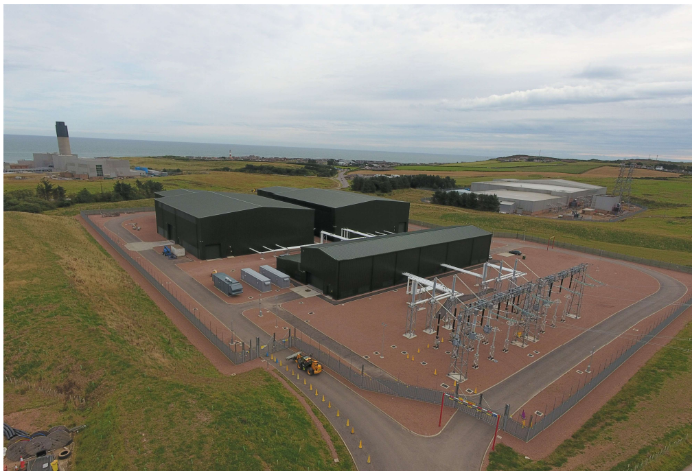
Plate 3-1 Example 400 kV Substation
