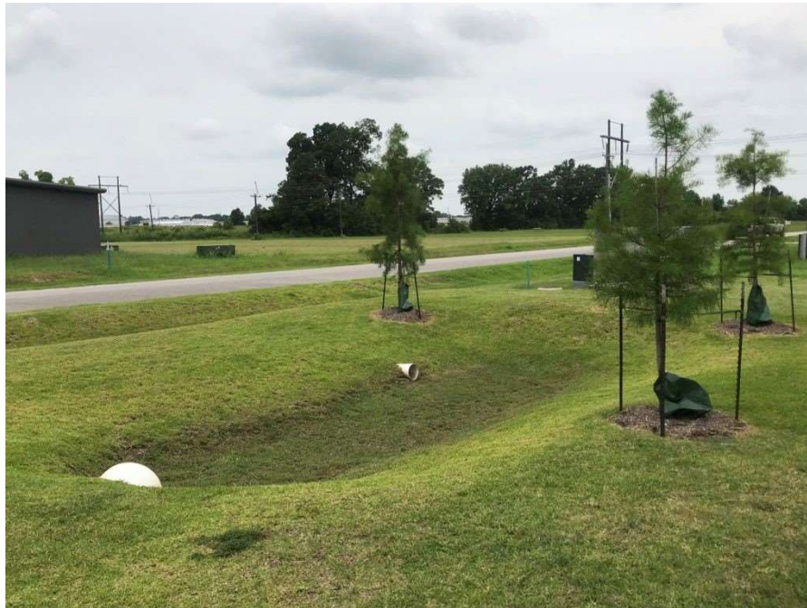
Plate 3-3 Example Small Detention Basin
