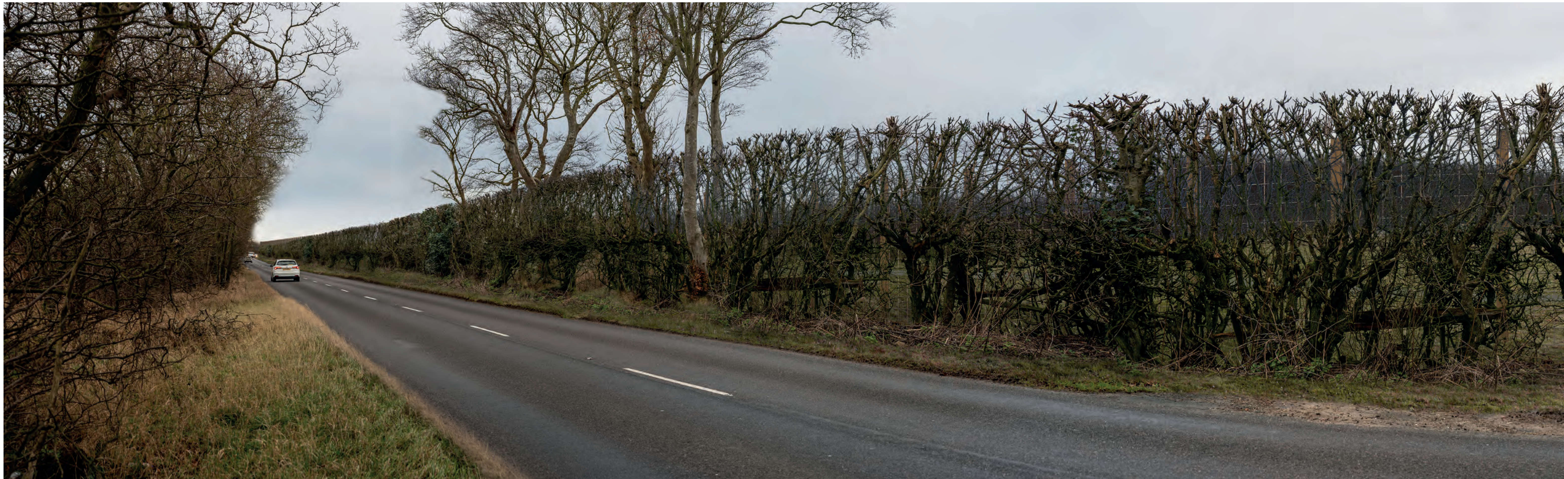
Viewpoint 1: Flushing, on A950 looking south: Sheet 16: View at Year 15
