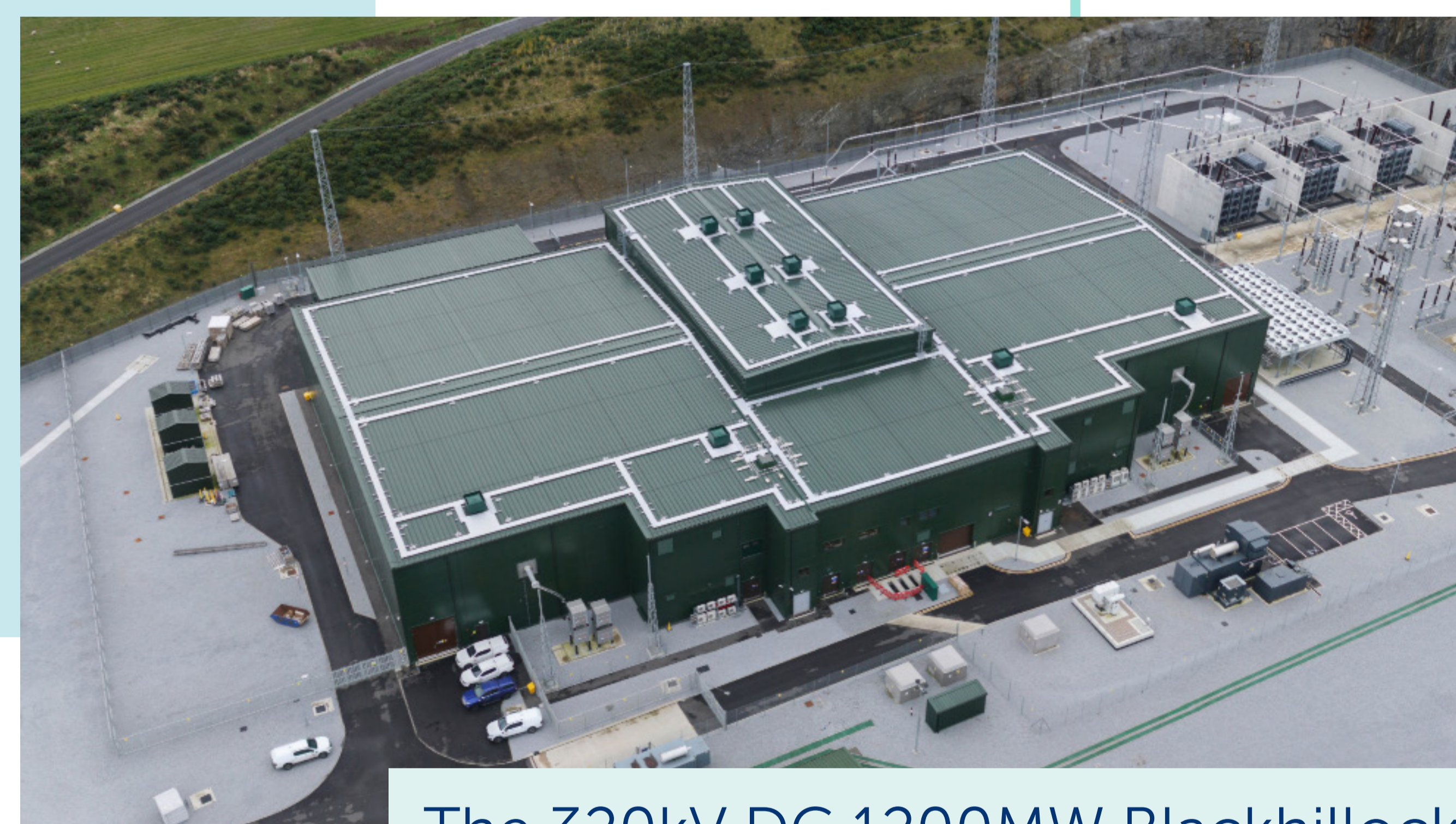
The 320kV DC 1200MW Blackhillock HVDC converter station.
