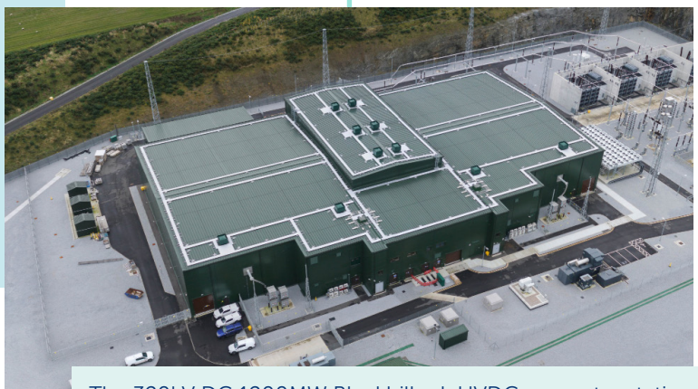
The 320kV DC 1200MW Blackhillock HVDC converter station
