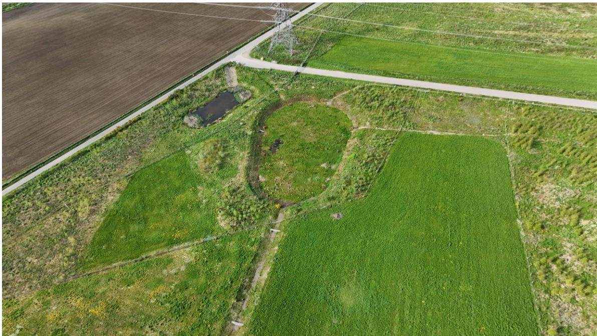
Plate 3-2 Example SuDS Basin
