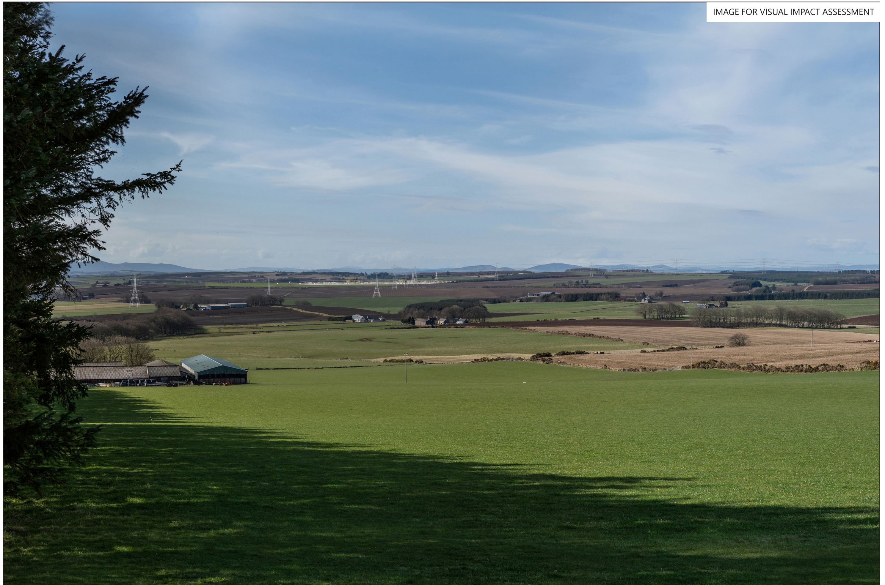
Greens 400 kV Substation Figure 8.10-e
