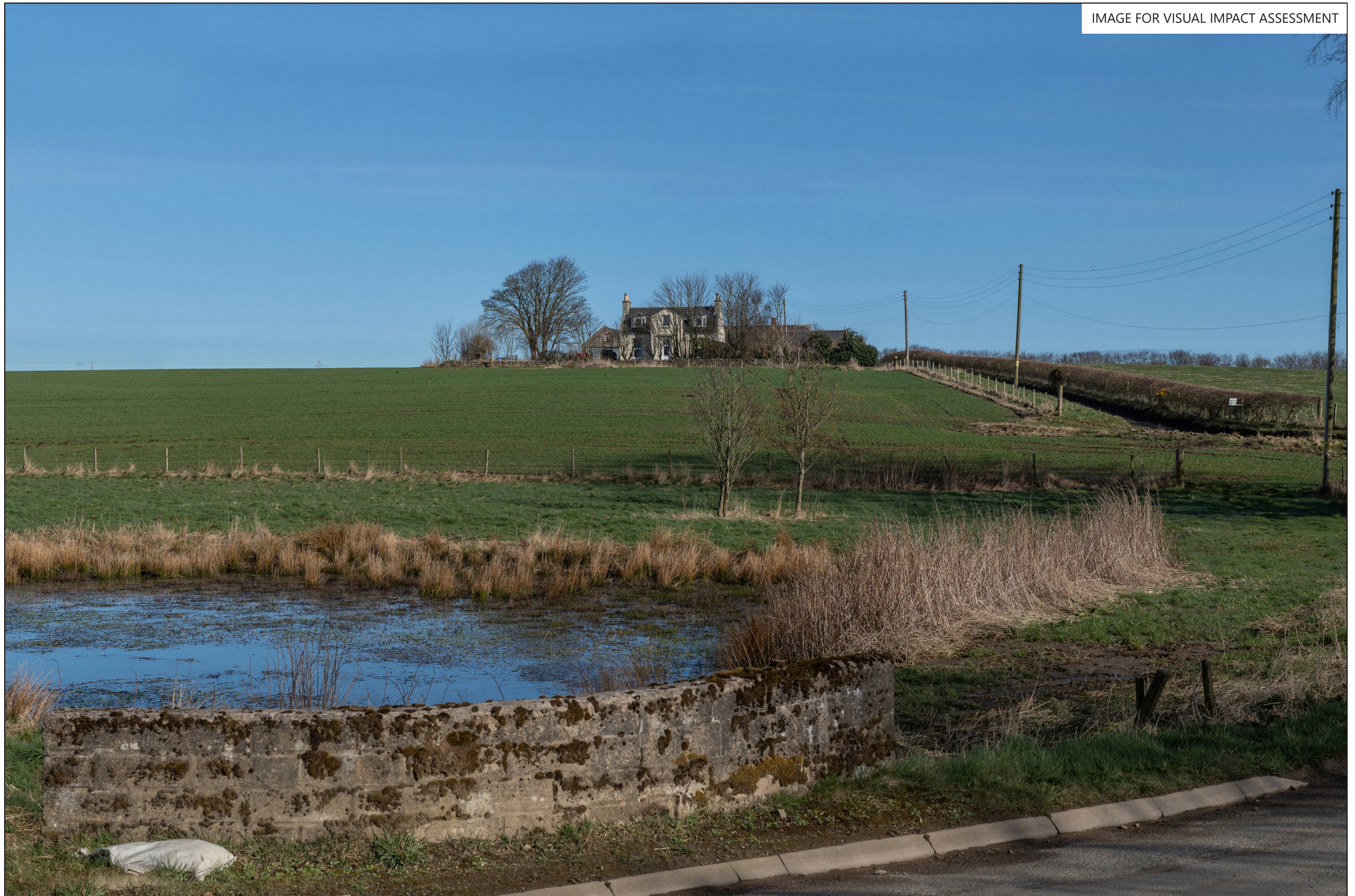
Greens 400 kV Substation Figure 8.16-e
