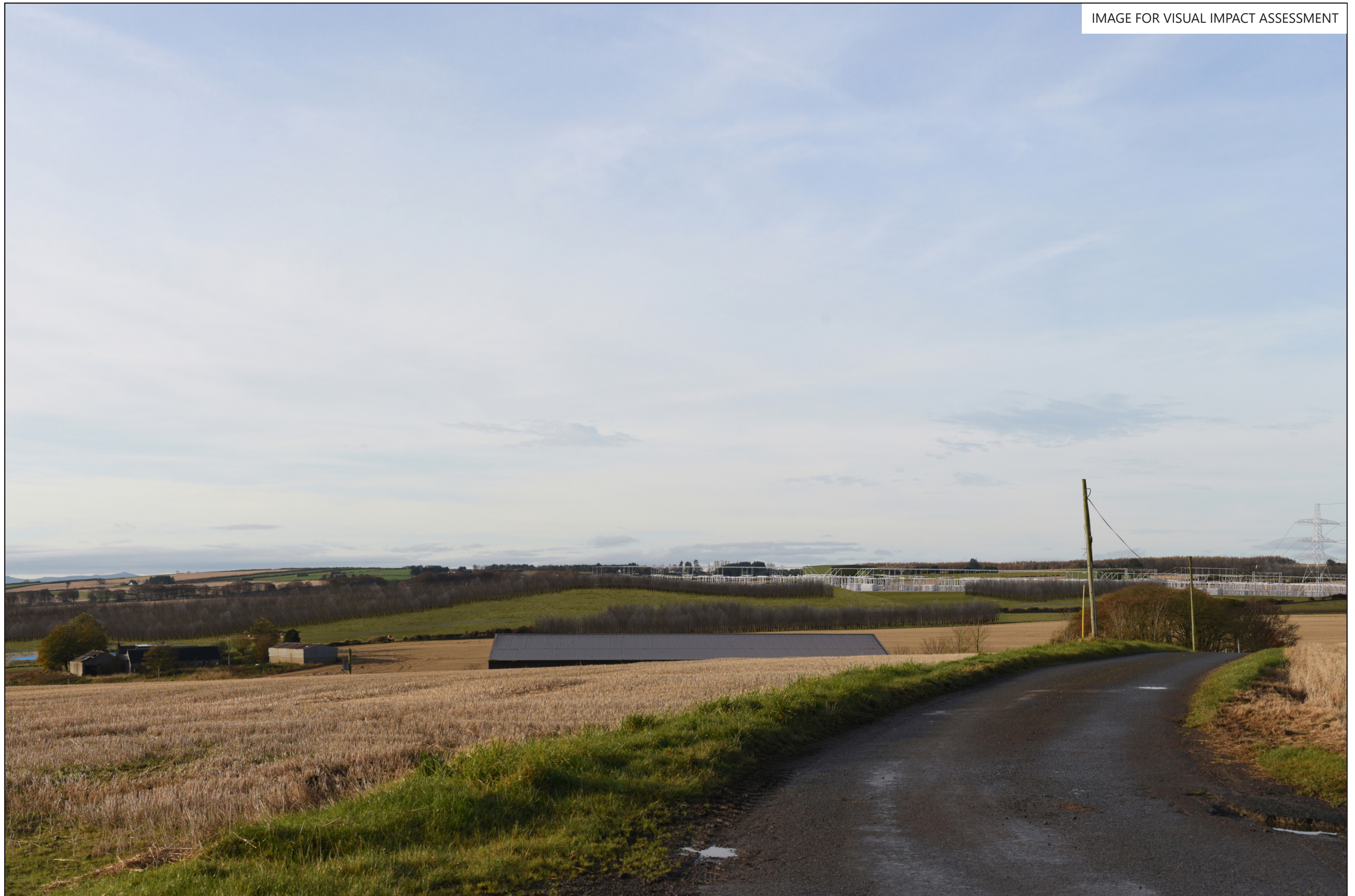
Greens 400 kV Substation Figure 8.9-f
