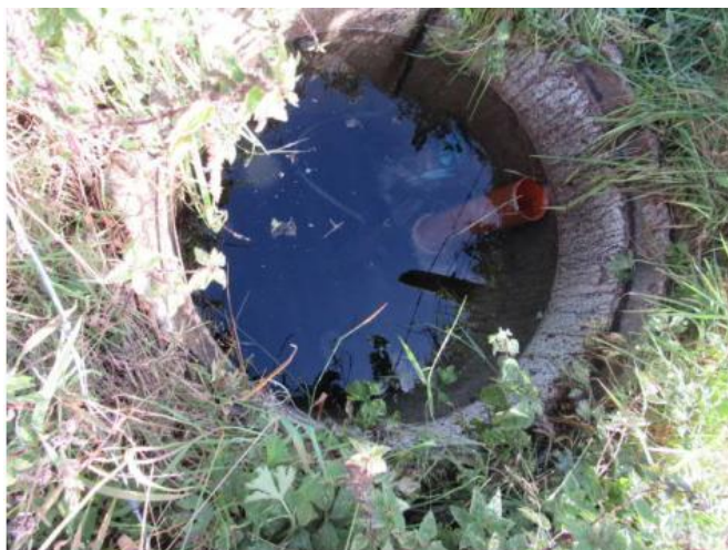
Photograph 7. Underground water supply tank (381534, 847532) within the Site (by walkover survey on 19 September 2023).
