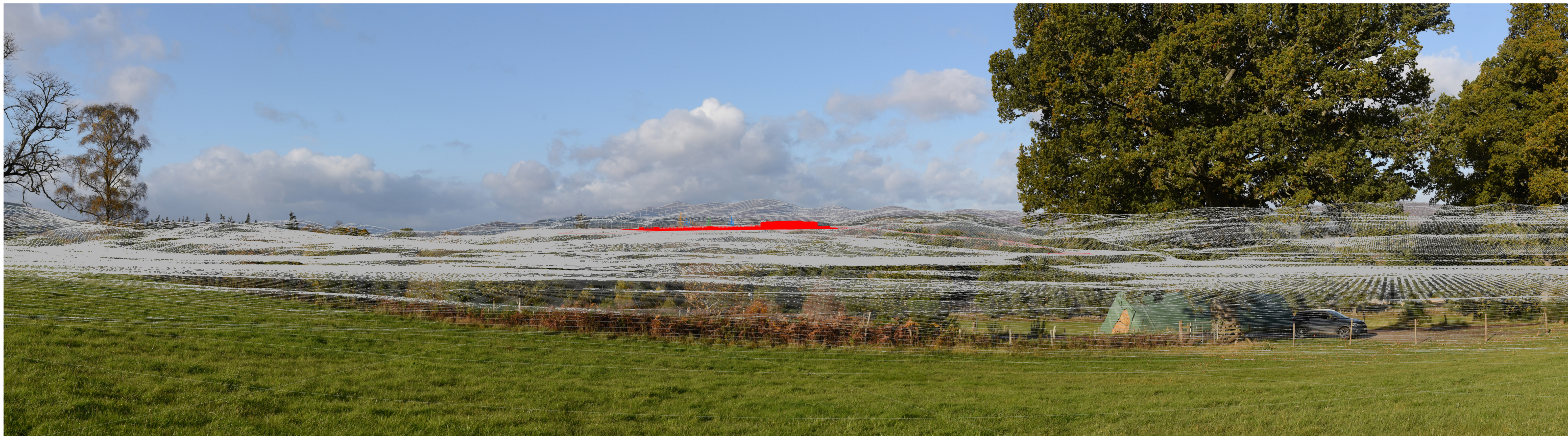
Figure 8.39b Viewpoint 14: View looking west from Belladrum Tartan Heart Festival Grounds Operational View (Photowire: Fanellan 400kV Substation & Converter Station & SSEN Cumulative Terminal Towers)
