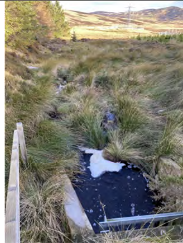
Photo 2.16: North looking after culvert
