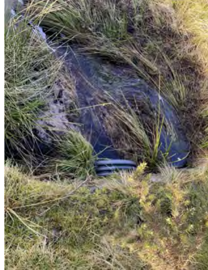
Photo 1.8: Culvert outflow (west facing)
