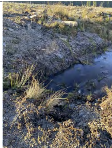
Photo 2.7: Ditch culverted under track (west)
