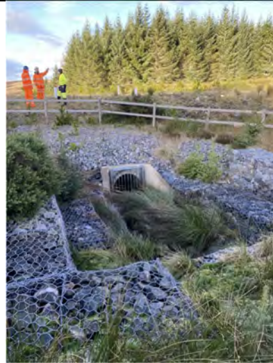
Photo 2.15: 1000mm culvert under substation access road
