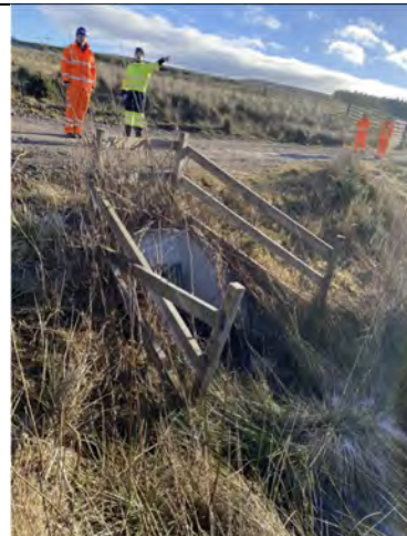
Photo 2.13: Substation surface water drainage enters ditch
