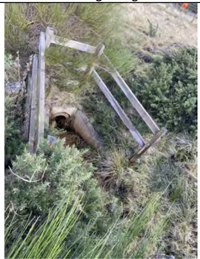
Photo 3.5: 225mm culvert under substation access road
