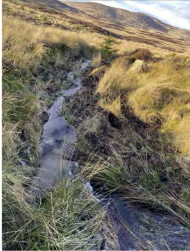
Photo 1.9: West looking downstream of culvert
