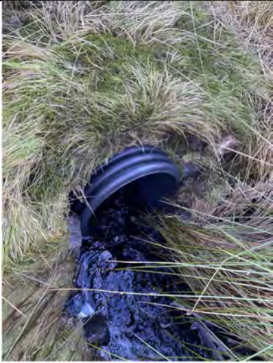
Photo 3.7: 450mm culvert under Lochbuie Road
