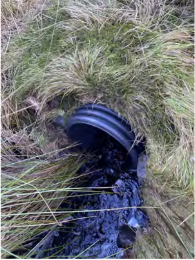
Photo 1.7: 450mm culvert under road
