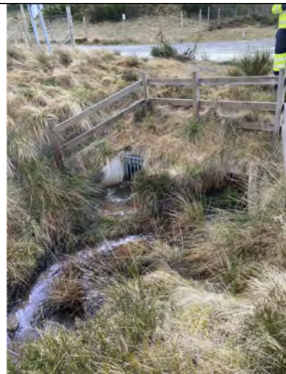
Photo 3.6: culvert outflow
