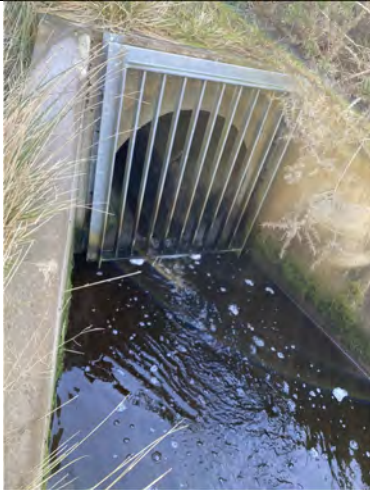
Photo 2.15: 1000mm culvert outflow
