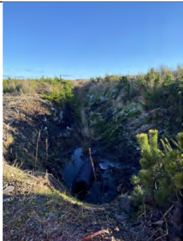
Photo 2.6: Ditch culverted under track (east)
