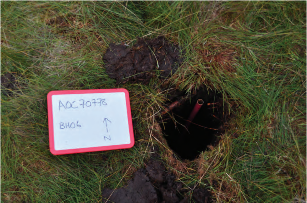
Plate 9: General view of BH06 post-excitation, looking north
