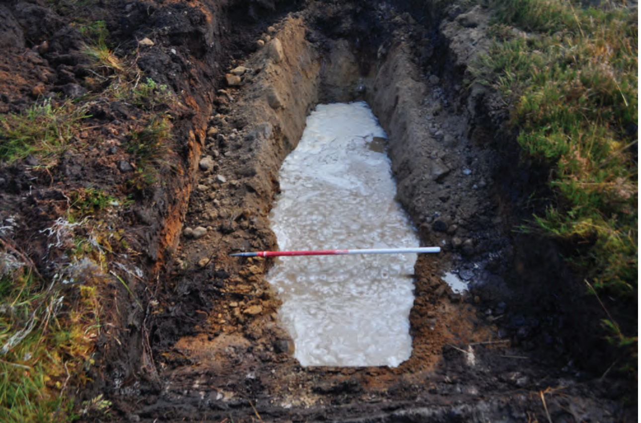
Plate 47: General view of TP21 soakaway during test, looking southeast
