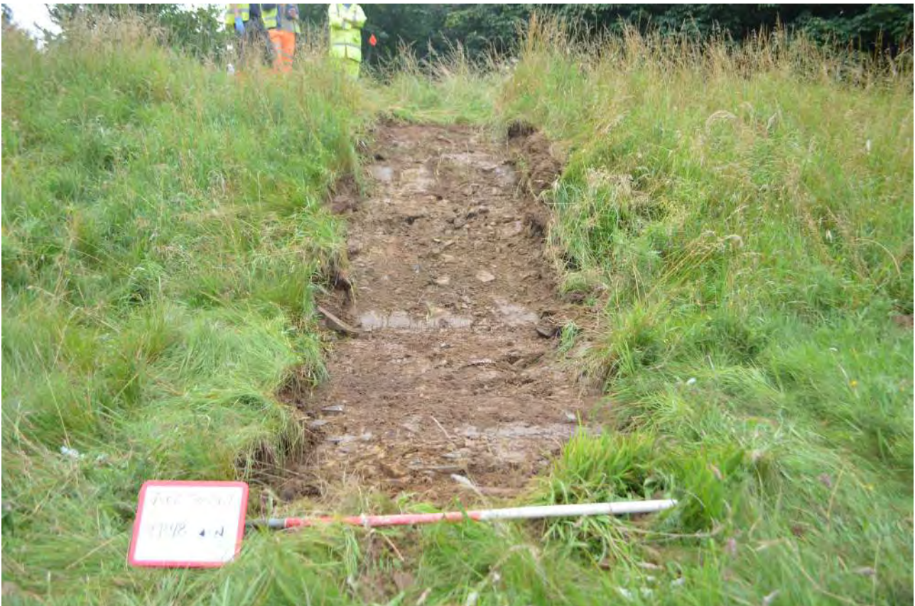
Plate 70: General view of TP40 down to rubble quarry backfill layer, looking east
