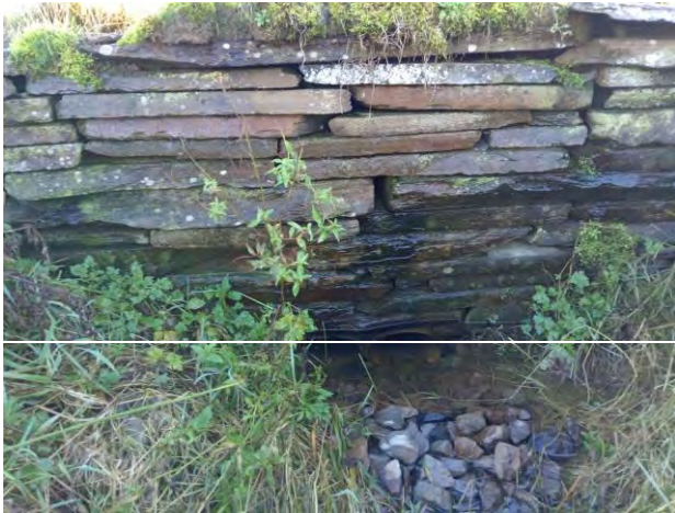
Photo 4.1 2 x 250mm Clay Pipes.
