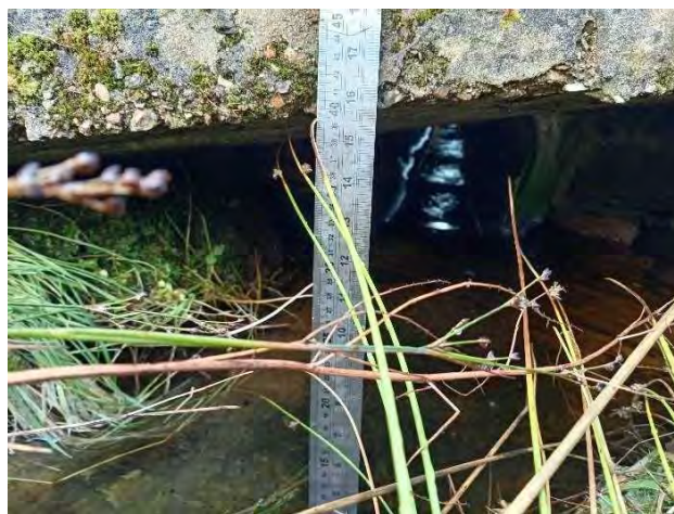
Photo 1.2 450mm Concrete Pipe Inlet
