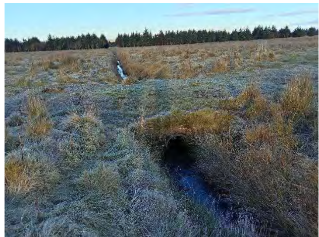
Photo 2.10 500mm Pre-Cast Concrete Pipe
