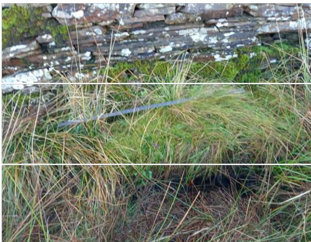
Photo 4.5 150mm Clay Pipe.
