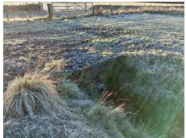
Photo 2.2 2 x 250mm PVC Pipe Outlet
