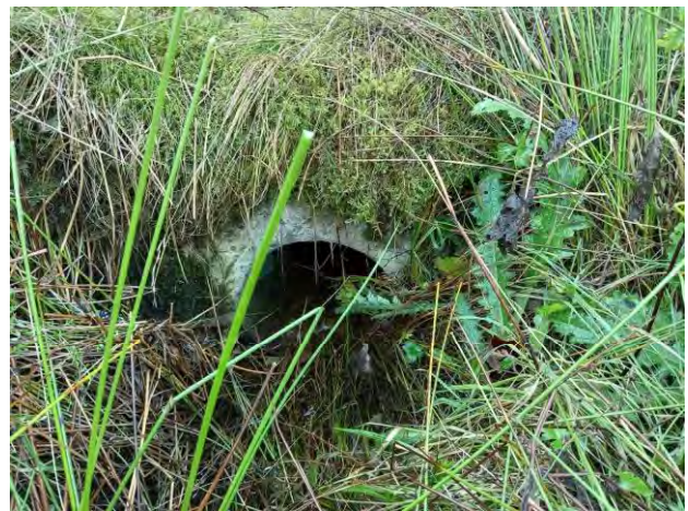
Photo 4.4 300mm Pre-Cast Concrete Pipe at A9.
