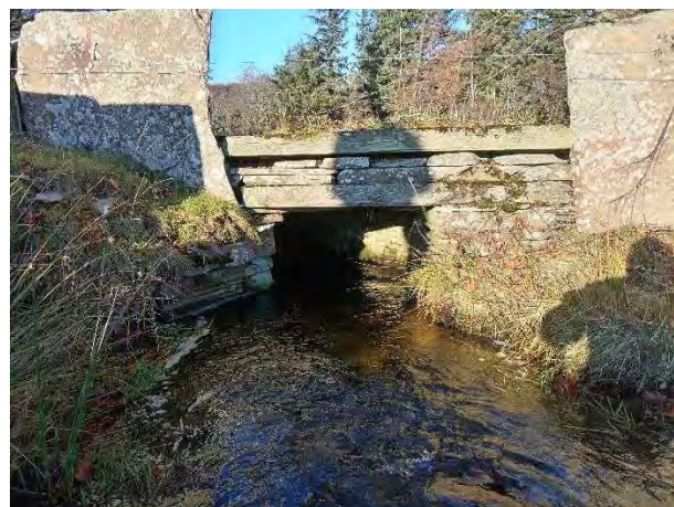
Photo 1.11 Masonry box culvert Upstream of Banniskirk House Access Road
