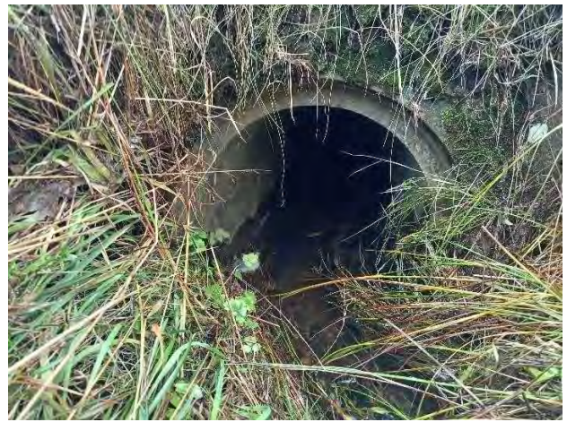
Photo 2.12 500mm Pre-Cast Concrete Pipe at A9
