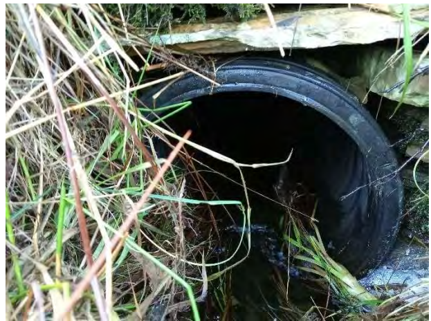
Photo 3.8 300mm Corrugated PVC Pipe at A9.
