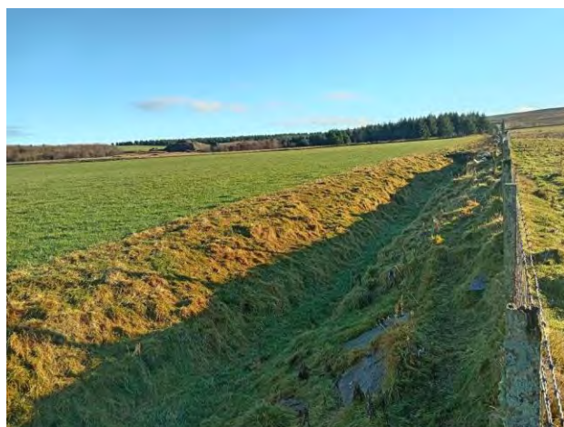
Photo 1.4 Downstream of Diversion Looking Upstream
