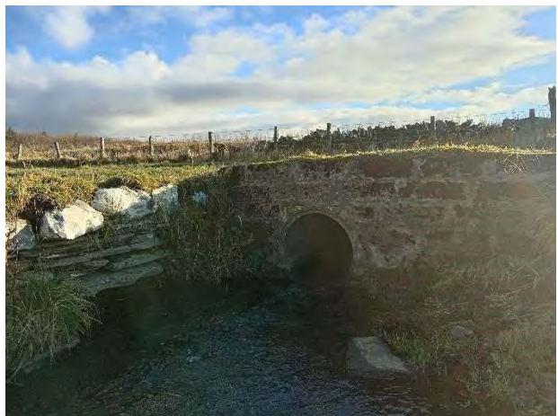
Photo 1.6 600mm Concrete Pipe Outlet
