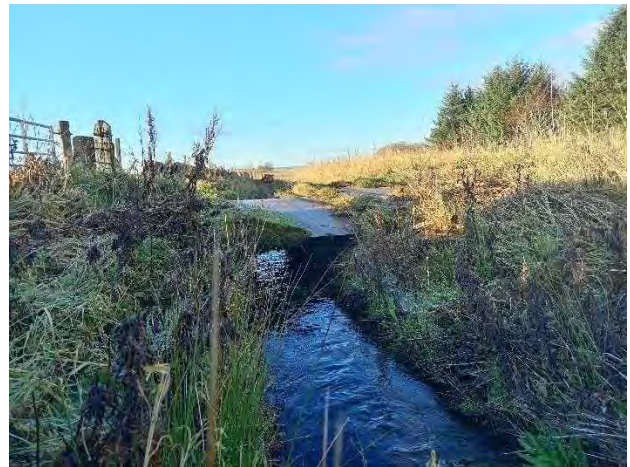
Photo 1.10 Masonry box culvert with sheet metal top
