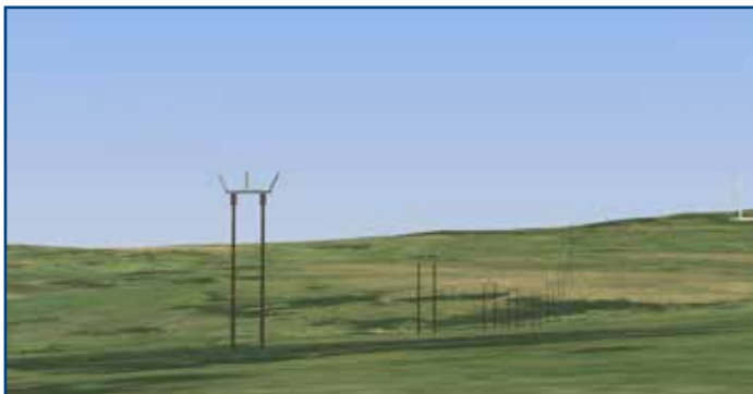
Figure 1 An Example of a Trident H wood pole structure
