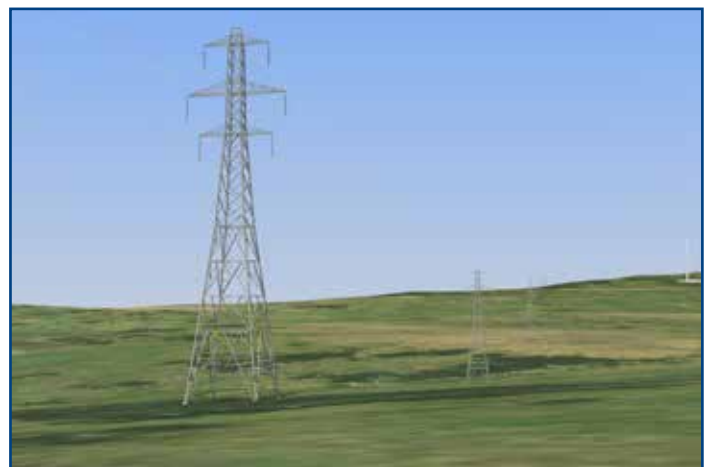
Figure 2 An example of a Steel Lattice Tower Structure
