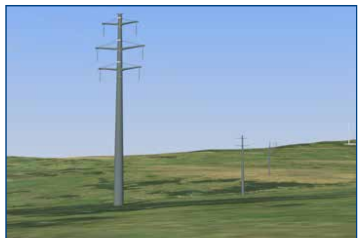
Figure 3 An Example of a NeST Steel Monopole Structure
