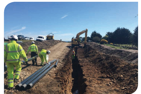
Duct trench for 132kV cable
