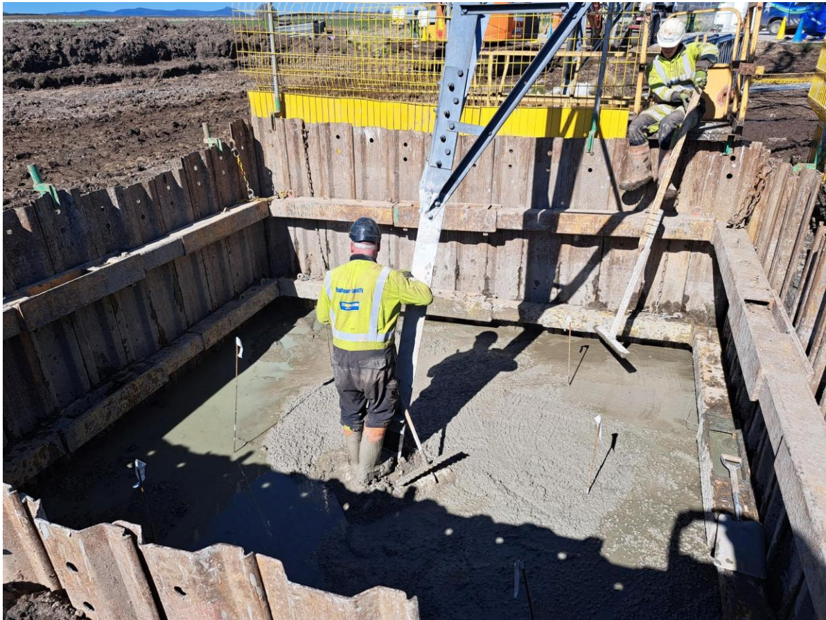
Plate V1-3.1: Illustrative Image of Tower Foundation Construction
