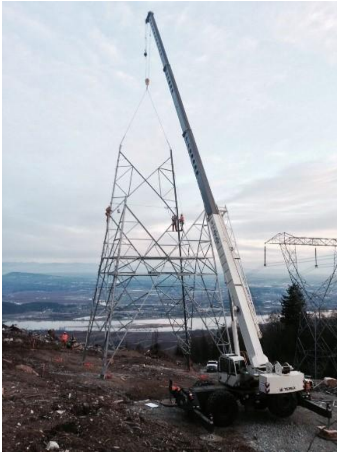
Plate V1-3.2: Illustrative Image of Steel Lattice Tower Construction
