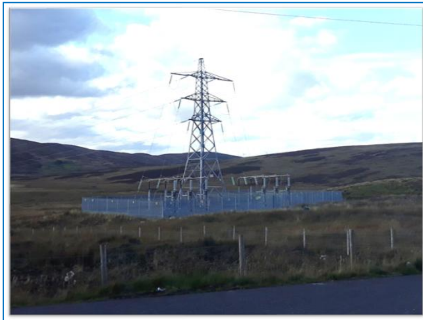
Plate V1-3.6: Example of a Cable Sealing End Compound
