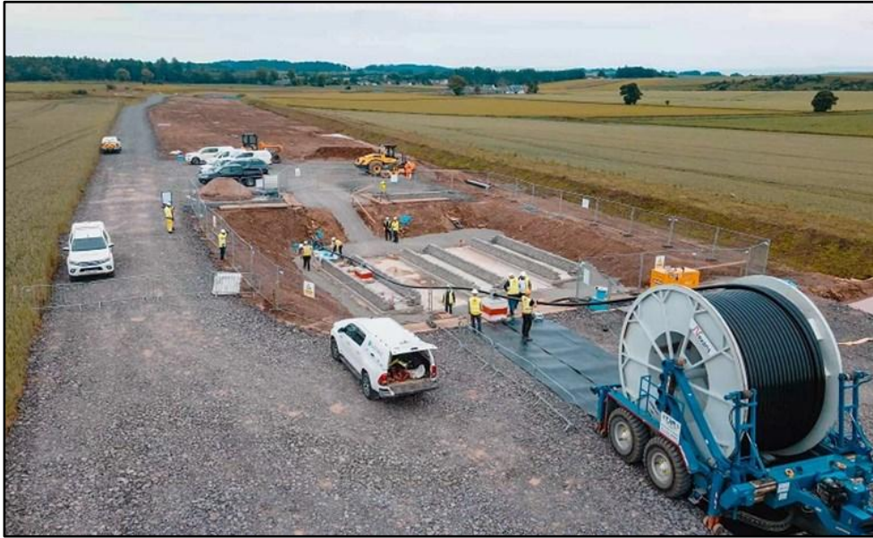
Plate V1-3.3: Photograph of Underground Cable Installation
