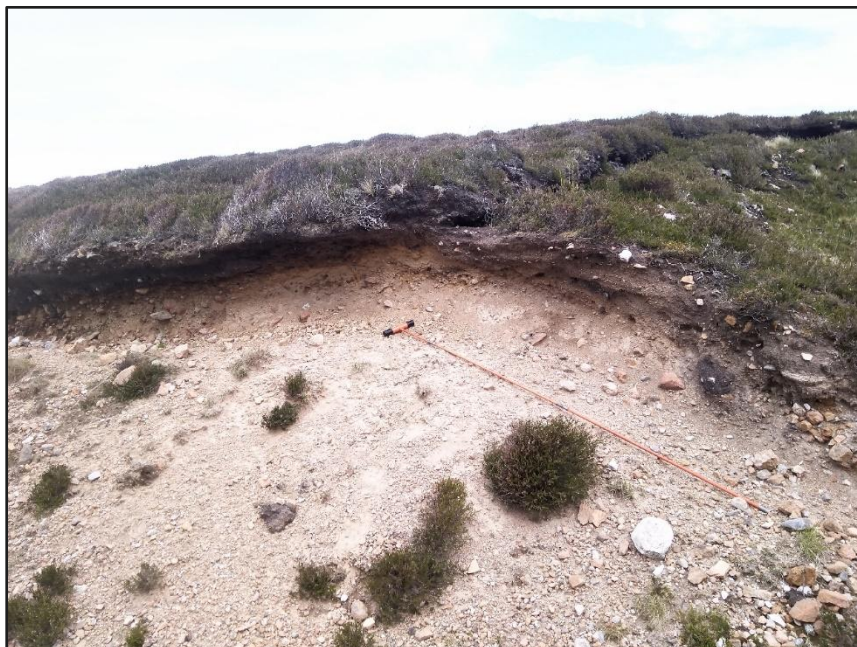
Photo 6: Road cutting displaying granular substrate at existing access track (to be upgraded) near Cnoc Eadar Dha Allt looking east. NGR: NC 86658 64682.
