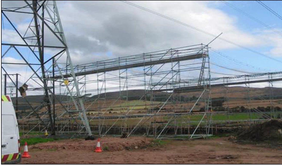
Photograph 3-4 Illustrative Image of Temporary Construction Scaffolds
