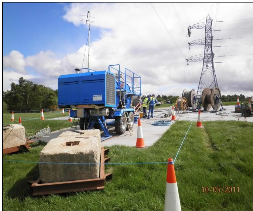
Photograph 3-2 Typical EPZ with equipment set up for reconducting
