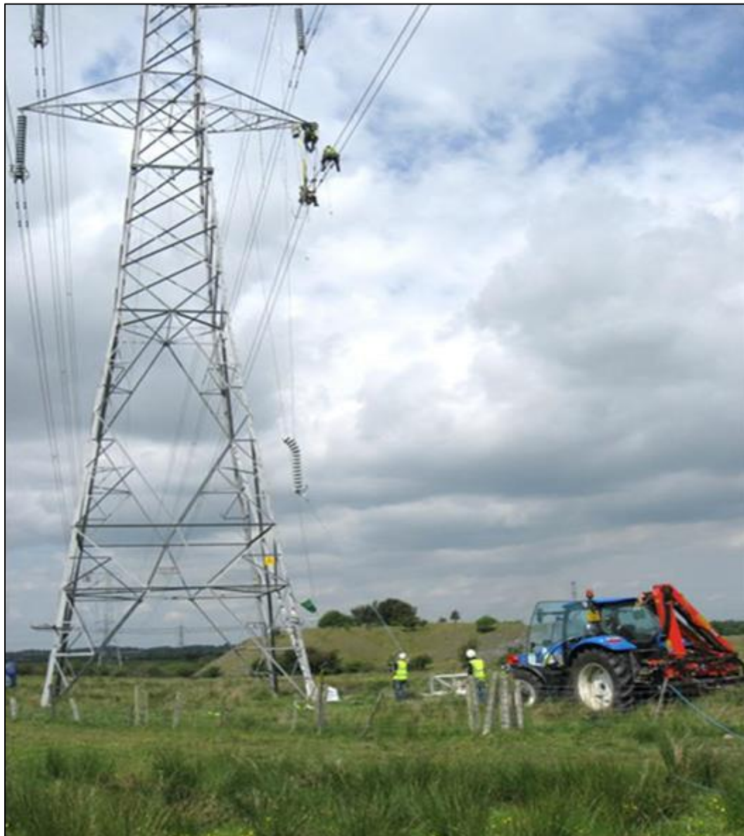
Photograph 3-3 Replacing insulators on an existing OHL tower
