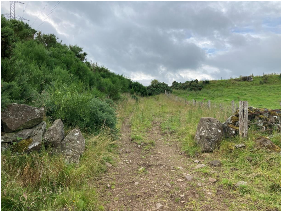
Photograph A11.2-25: View of existing track where a 'Bespoke Track' is proposed to provide access to Tower 66 showing existing break in drystone wall on the northwest side of Colzie Hill.
