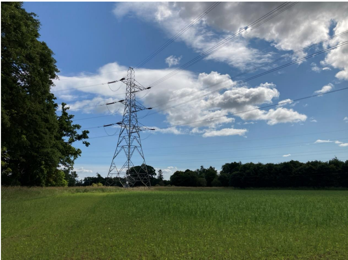
Photograph A11.2-16: View of Tower 115 from the west with woodland that forms part of Megginch GDL (GDL00278) will be subject to crown reduction and limited tree loss (inline with the OHL resilience works).
