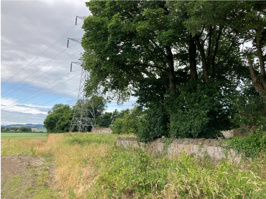
Photograph A11.2-20: View west to Tower 97, an area where access is proposed via 'Trackway Panels'. Pitfour Walled Garden (MPK18871) located to the right of the image.
