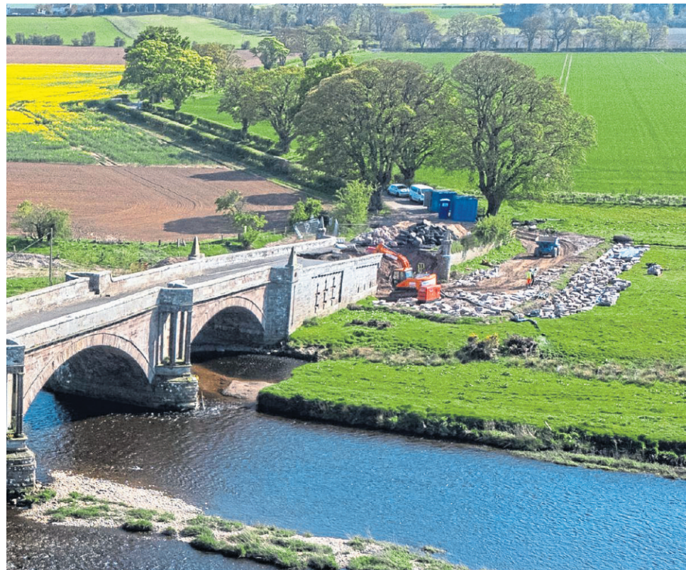
AERIAL VIEW: Drone footage of the repair work being carried out at Bridge of Dun, near Montrose, after it was damaged during Storm Babet. Picture by Kim Cessford.
