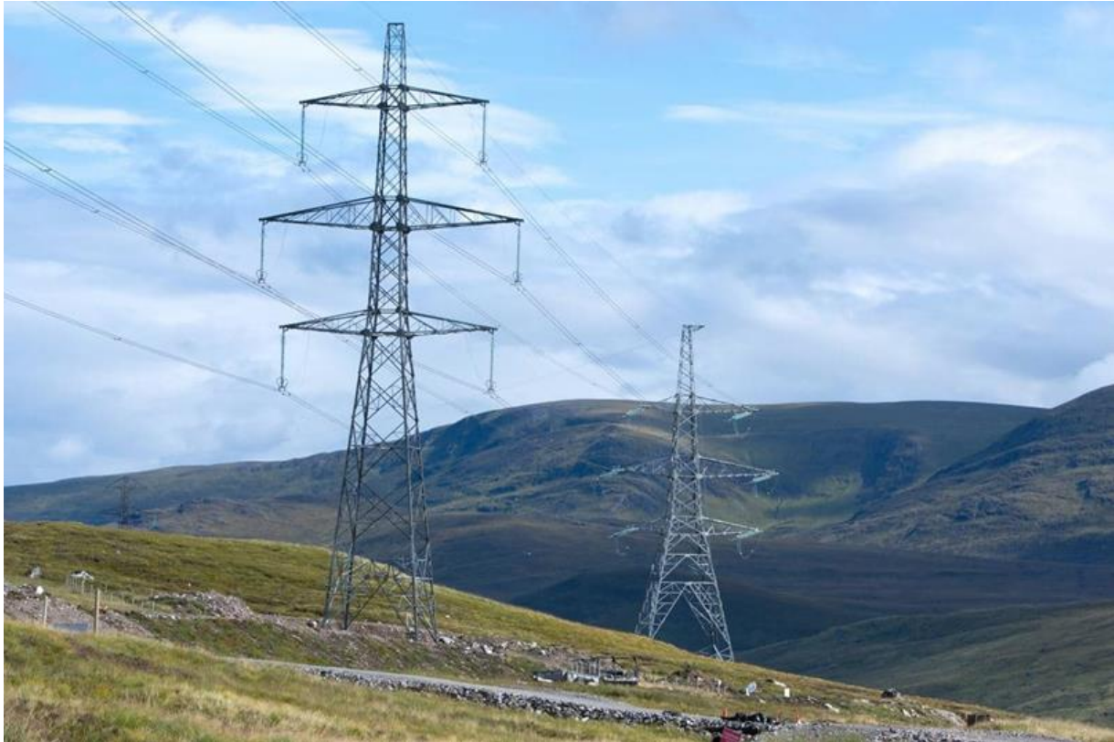
Plate 2.1 – Existing SSE400 steel lattice tower design
